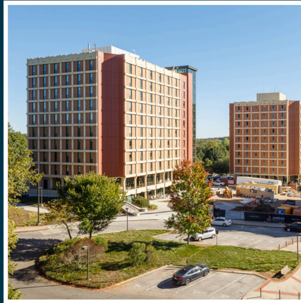
CLEMSON UNIVERSITY BYRNES HALL Student Housing Renovation
